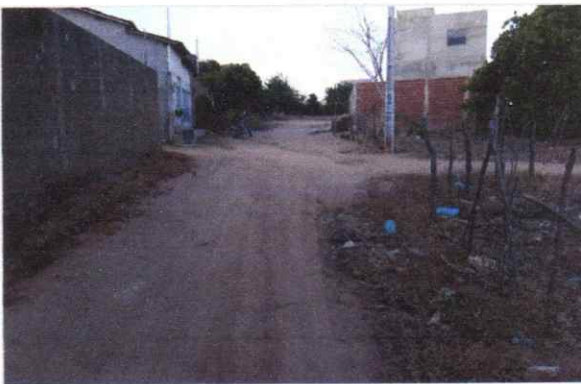
RUA PROJETADA II - FINAL 24 M 615940.79 m E / 9324141.48 m S
